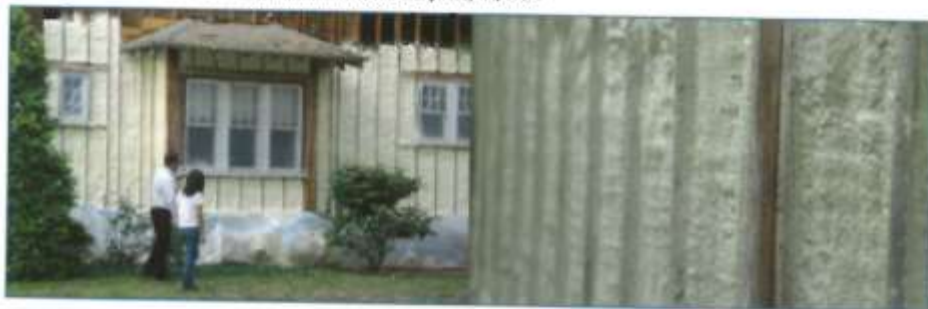
▼ Fig. 6: Pictures of foam application in West Lafayette, IN, USA
