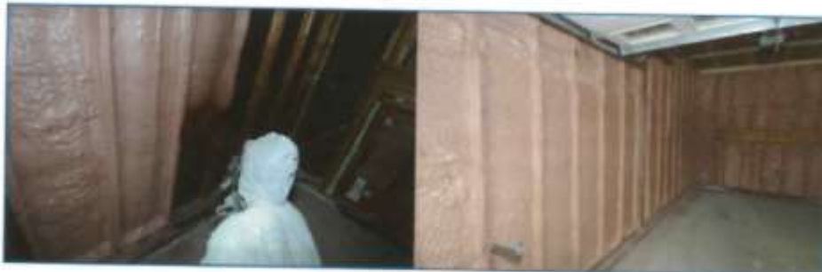
▼ Fig. 7: Pictures of foam application at second application area
