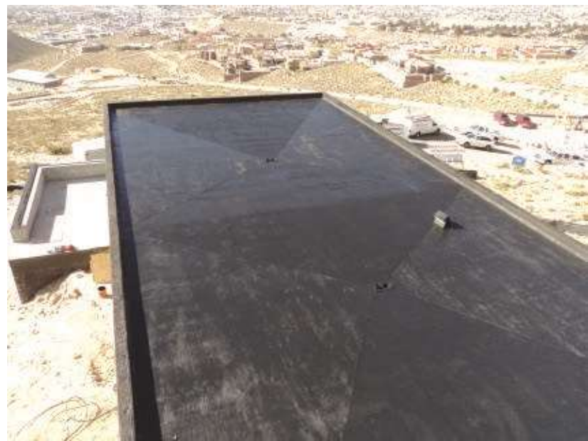
Top: View of the upper roof of the house;
