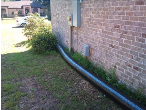
Figure 31 Direct exhaust to a safe location
