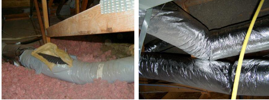
Figure 15 Ductwork should not be damaged during the SPF application process
