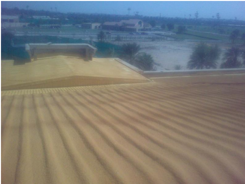
Figure 3 SPF offers seamless insulation
