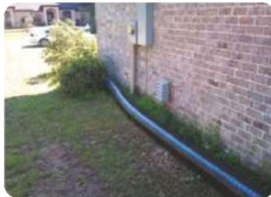
Figure 31 : Direct exhaust to a safe location
