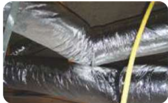
Figure 17 : Ductwork should not be damaged during the SPF application process
