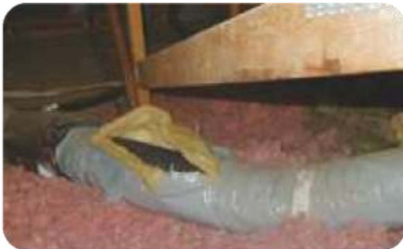
Figure 17 : Ductwork should not be damaged during the SPF application process
