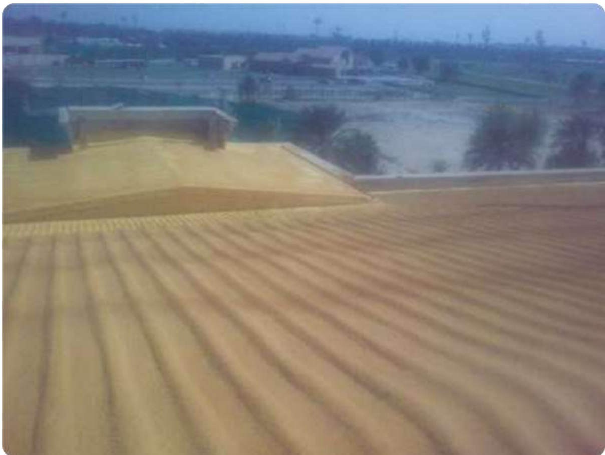
Figure 5 : SPF offers seamless insulation
